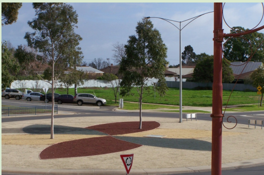
Gravel Mulch Treatment Roundabout Swan Hill
