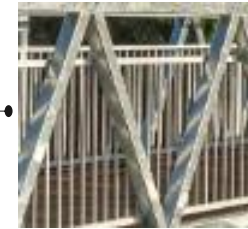
Galvanised Steel Trusses: Equal Angles – cleats connections
