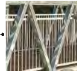
Galvanised Steel Trusses: Equal Angles – cleats connections
