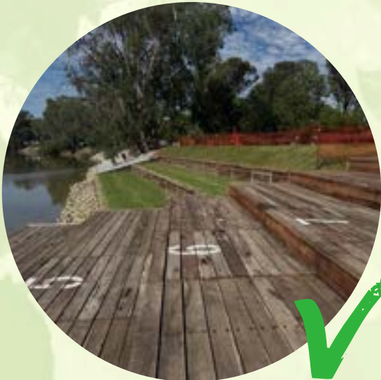
Swan Hill Ten Steps replacement and three-tiered retaining wall
