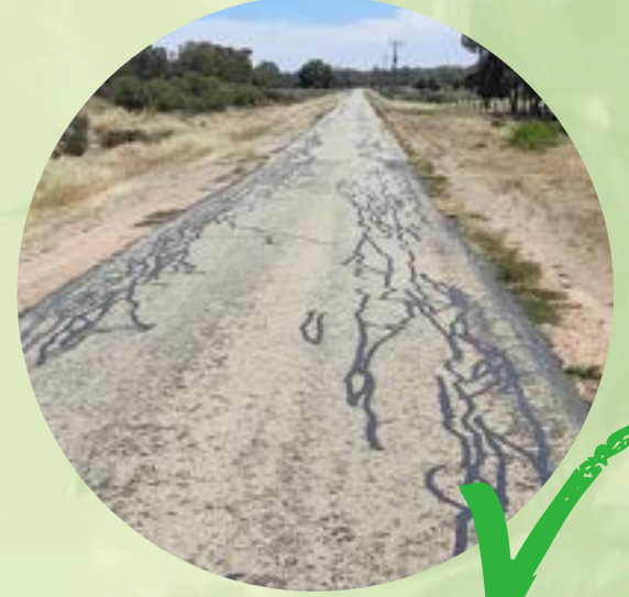
Crack sealing - Murraydale Road
