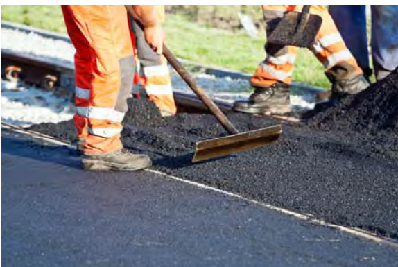
Gravel Re-sheeting & Road Reconstruction of roads
