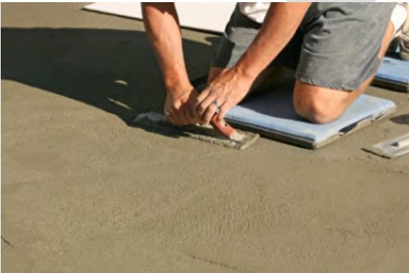
Concreting of major footpaths
